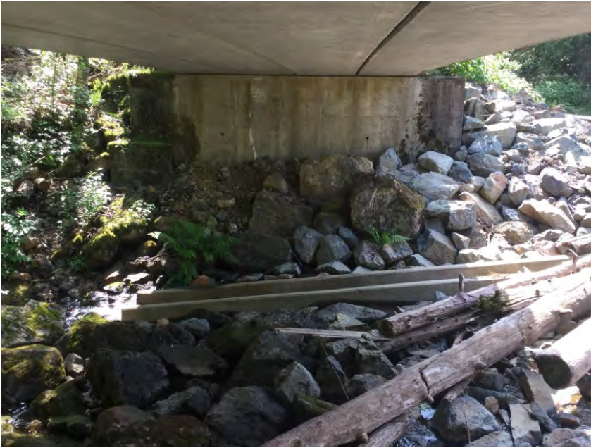
Right Bank Abutment when facing downstream
