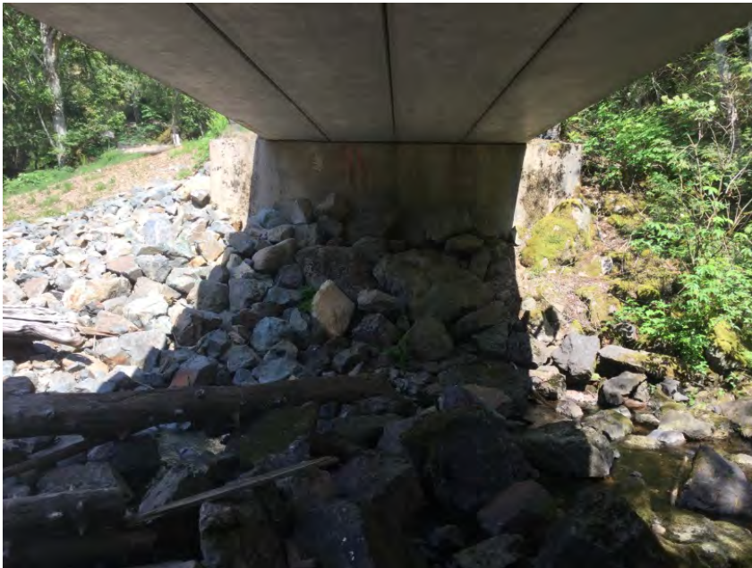
Left Bank Abutment when facing downstream
