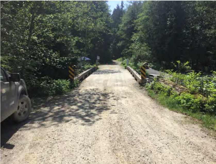
Approach from Left Bank when facing downstream
